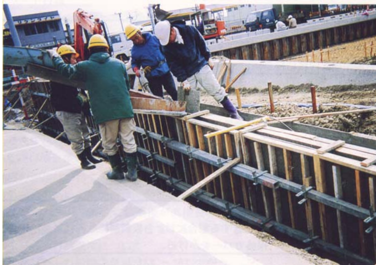
Under construction for channel
