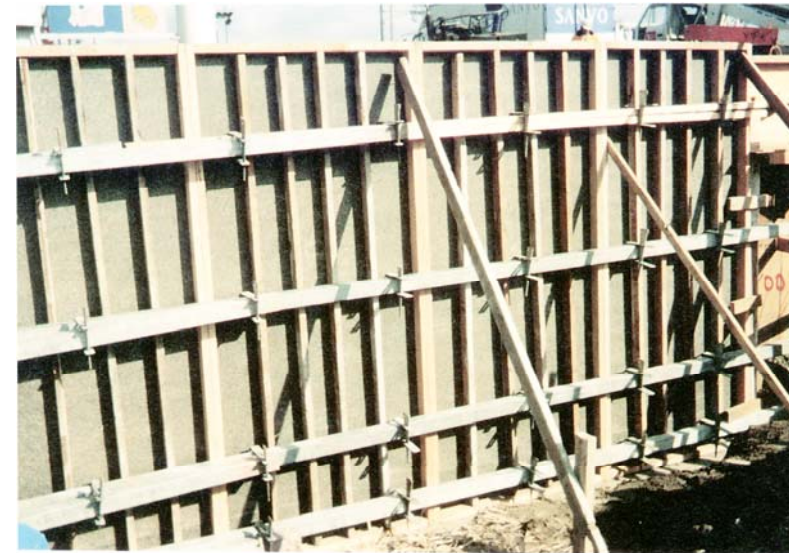
Concrete form panels at construction site
